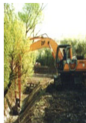
Land Drainage Works
